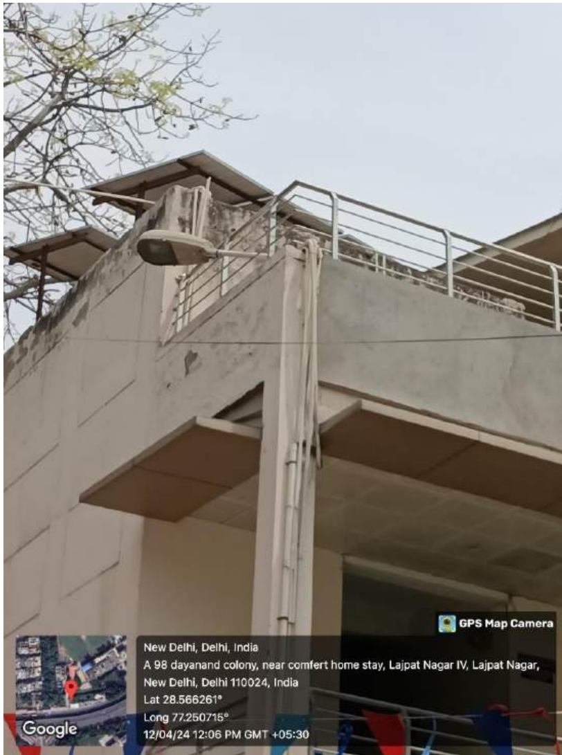
Fig III. 3 : Solar panels at rooftop of PGDAV college
